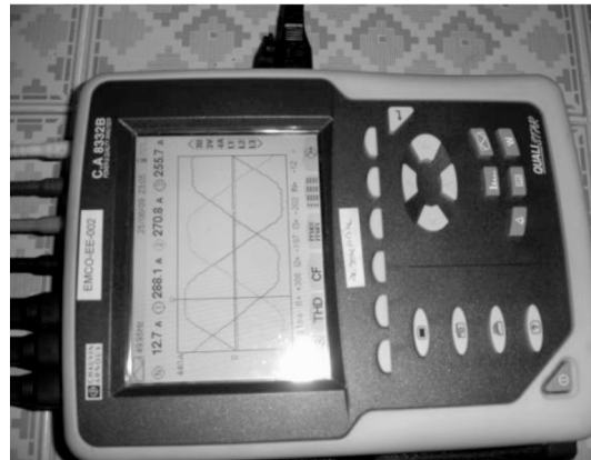
Figure 9 The installing of Equipped with measuring consumption
