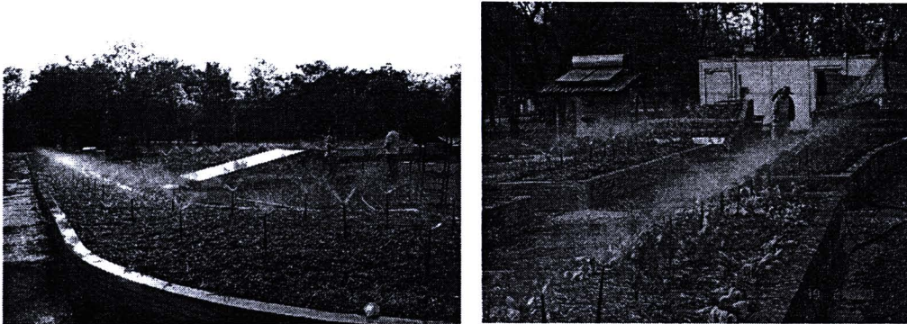
Figure 15 Sprinkler System Project at SERT
