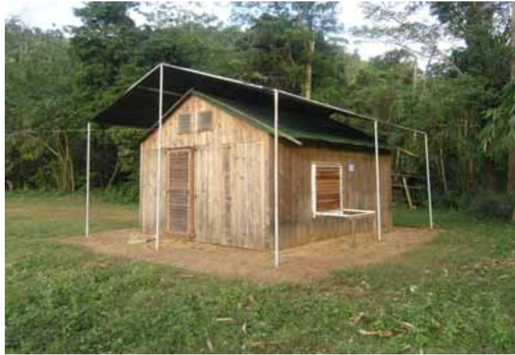
Figure 6 Hut frames from iron pipe and custom-welded galvanized pipes
