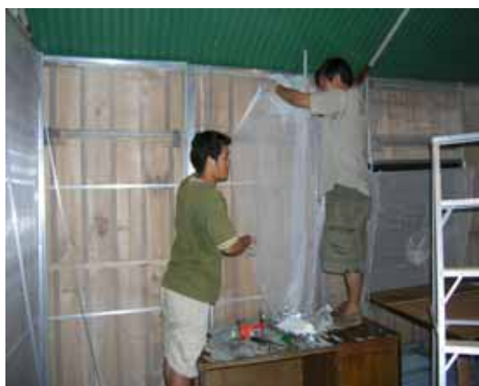
Figure 9 A series of panels were developed for holding treated netting which could be positioned around the interior surface of the hut
