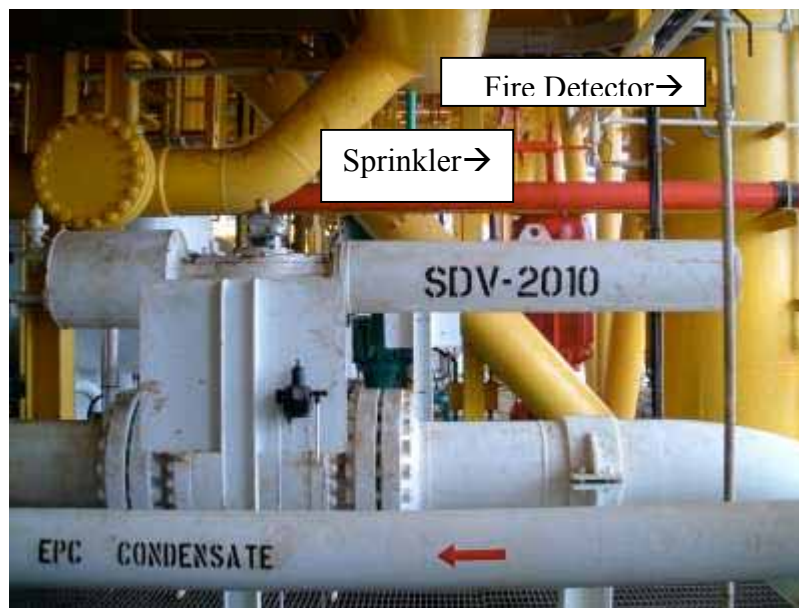
Figure 11 UV Detector and Sprinklers
