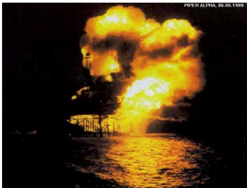
Figure 7 Piper Alpha, Major Explosion when the risers burst, the resulting jet of fuel dramatically increased the size of the fire from a billowing fireball to a towering inferno.
