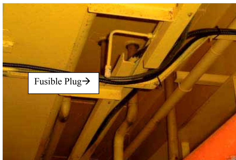
Figure 10 Fusible Plug at the PESDV location
