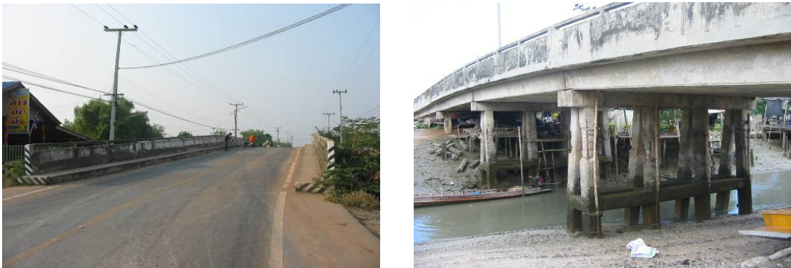
Figure 25 Example of concrete bridge to investigate
