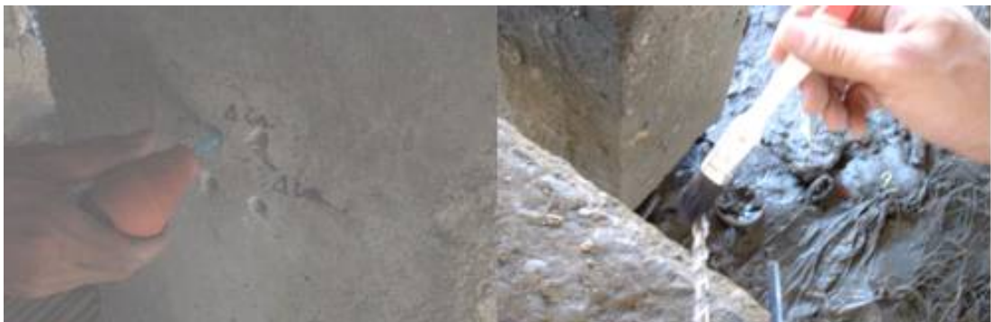
Figure 32 Clean the hole and drill before drilling next level
