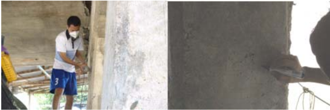
Figure 30 Clean surface and marking of location to drill
