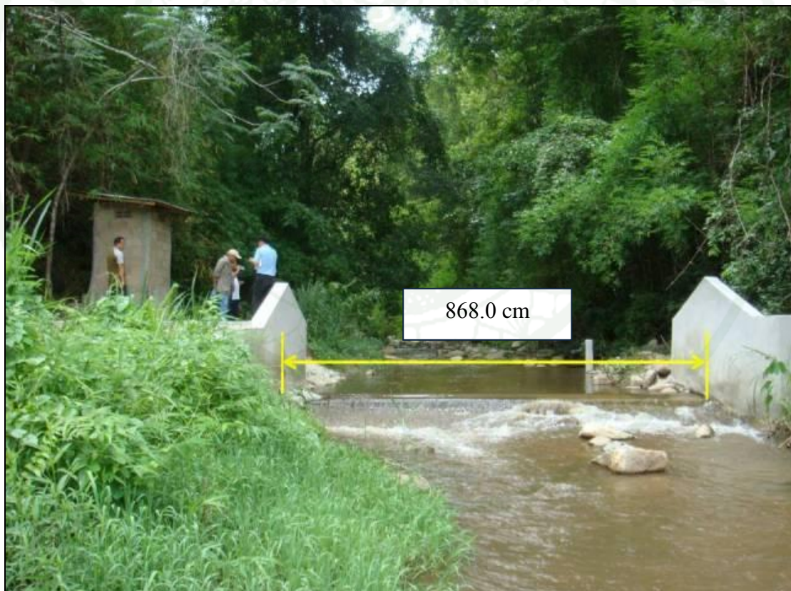
Appendix Figure 2 General Drawing of Mae Sai Weir (top) and picture of weir (below) at the outlet of Huai Mae Sai.
