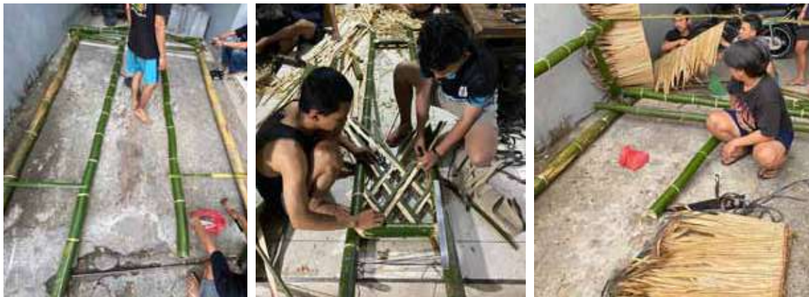
Figure 8. (Left) Making the structural posts of the Baruga, (Center) Weaving the Baruga walls, (Right) Installation of the Baruga roof use Nipa leaves.
