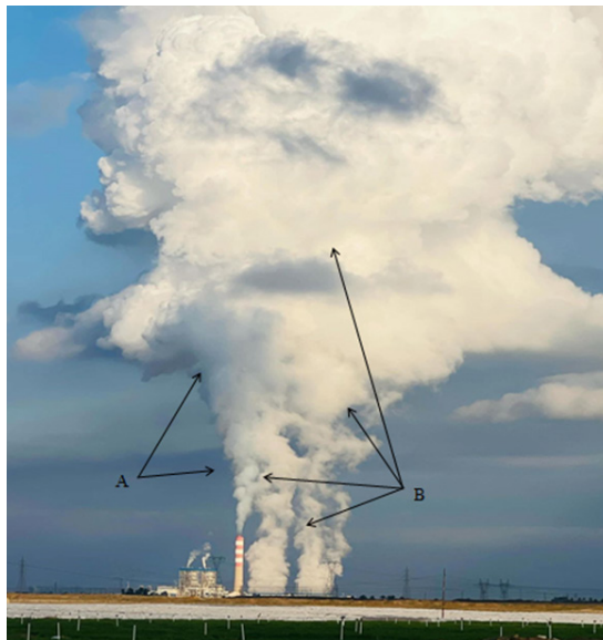
Figure 2. Represent all gas exhaust from Salah Al-Din thermal power plant. A-Smoking emissions from power plant produced from burning fossil fuel used to boil water in boilers. B-Evaporation produced from condensers into the atmosphere.
