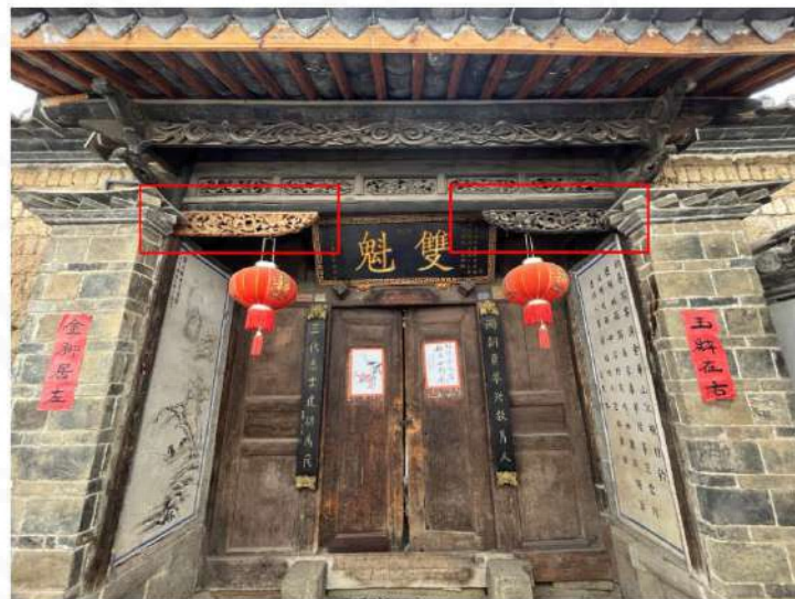
Figure 10 Restoration of Queti on the gates of a Ming Dynasty dwelling.
