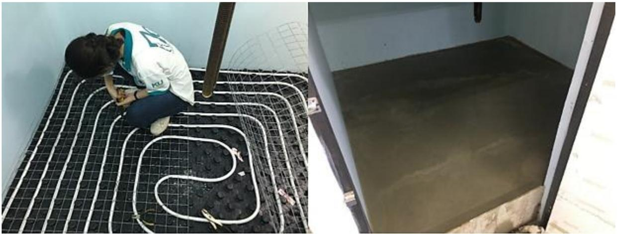
**Fig. 1.** The radiant floor cooling installation.
