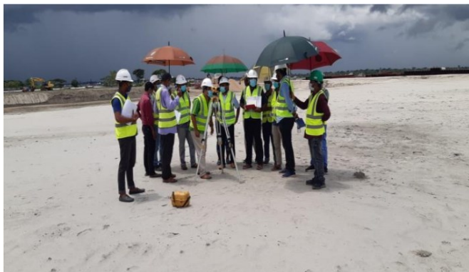
Figure 12 Taking the settlement plate reading
