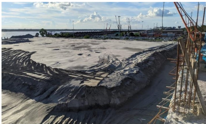
Figure 11 At the final height of the preloading level
