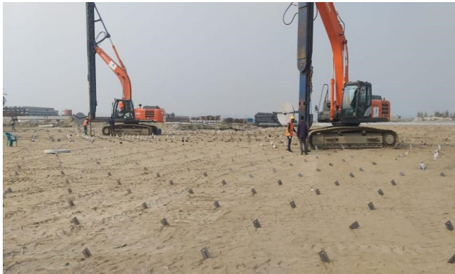
Figure 10 PVD driving at a triangular pattern
