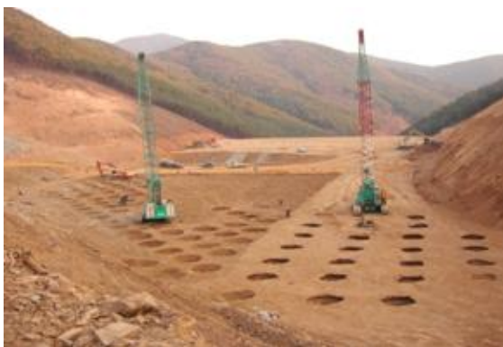
Figure 1.2 Scene of dynamic compaction
