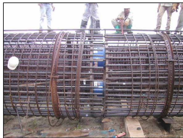
Figure 6. Assembling of O-Cell Jacks
