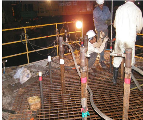
Figure 9. The Operation of Cracking Work
