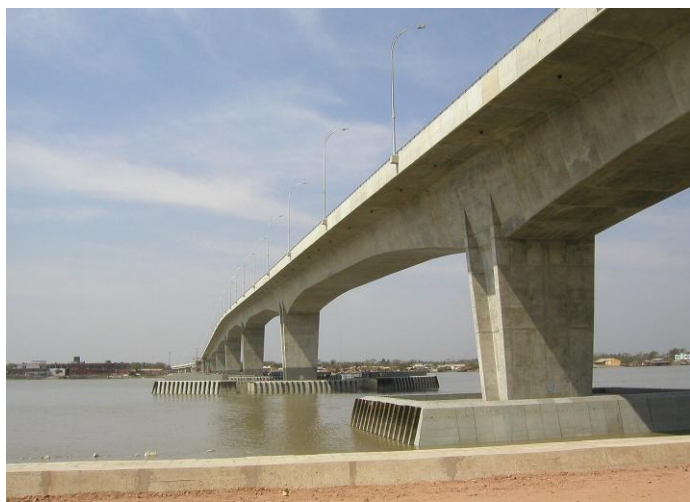
Figure 11. Main Bridge General View from North West side (2005)
