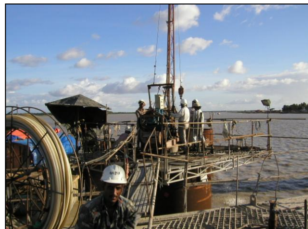
Figure 10. The Last Shaft Grouting at MP4
