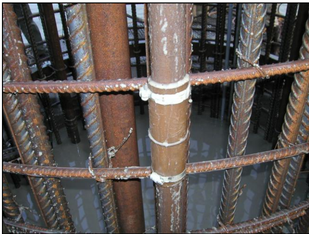
Figure 3. Fixture of TAM pipe on Pile Cage
