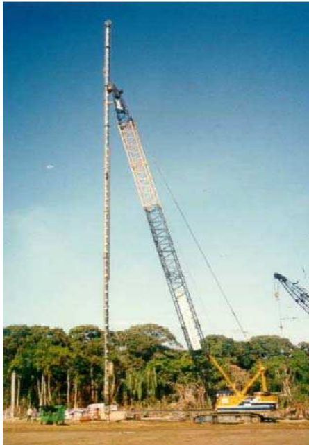
Fig. 7 A 50m-vertical drain installation at Miri
