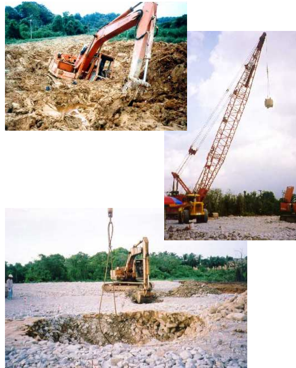
Fig. 28 Site condition before treatment (top); 300 ton.m DR rig (middle) and 3.5m diameter DR rock column (bottom) at Senai.
