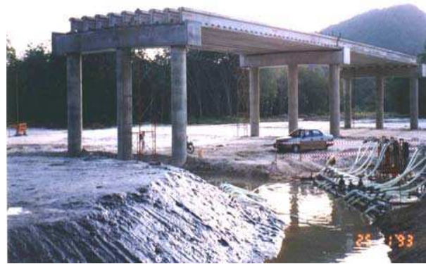
Fig. 10 Vacuum consolidation for the North-South Expressway in Ipoh
