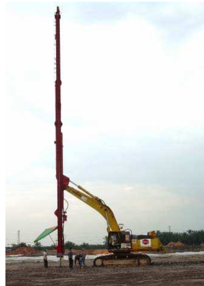
Fig. 8 Installation of vertical drains using hydraulic rig.
