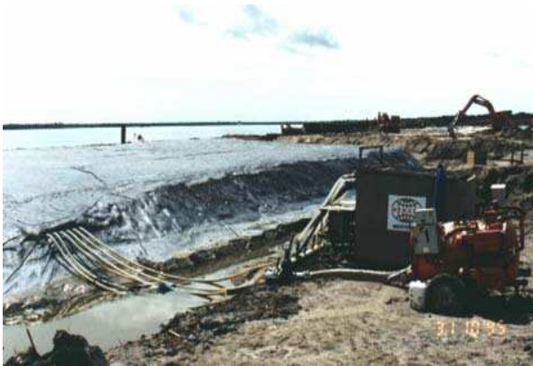
Fig. 12 Vacuum consolidation for the New Kuching Deepwater Port at Kg. Senari, Sarawak
