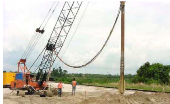
Fig. 19 Electric vibroflot for sand compaction
