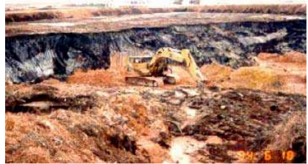
Fig. 1 Excavation and replacement of unsuitable materials
