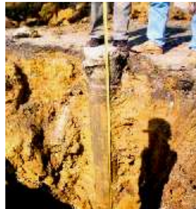
Fig. 31 Cross-section of raised embankment (top) and trial column (bottom) at Sebubut Dam.
