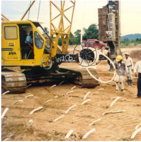
Fig. 4 Installation of cylindrical vertical drains in Ipoh for the North-South Expressway
