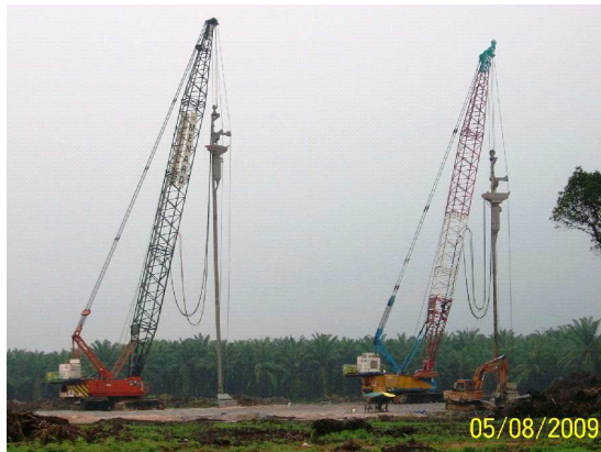
Fig. 26 Dry bottom feed stone column installation at SKVE
