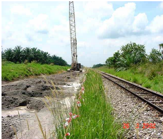
Fig. 17 SVC using dynamic compaction at Bidor-Kampar for the Rawang – Ipoh Double Tracking project
