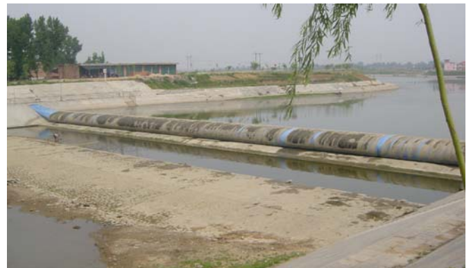
Figure 1. A rubber dam crossing a river
