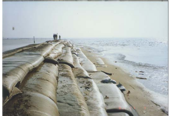
Figure 4. Dike constructed using clay slurry filled geosynthetic mats
