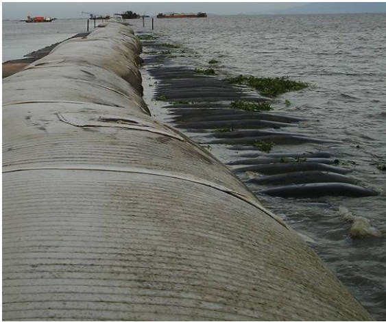
Figure 2. Use of sand filled geotextile tubes for shoreline protection in Malaysia (after Lee, 2009)
