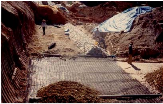
Figure 10d Rehabilitation in progress, 1989
