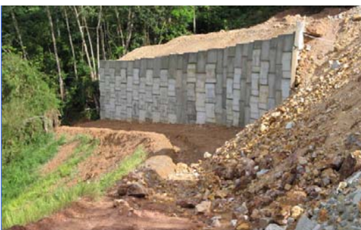
Figure 20b Anchored soil wall completed on 21 st May 2006
