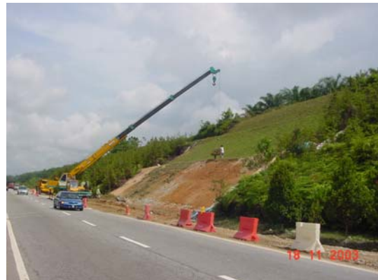
Figure15d Rehabilitated slope
