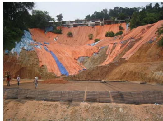
Figure 20i Construction of upper geogrid embankment
