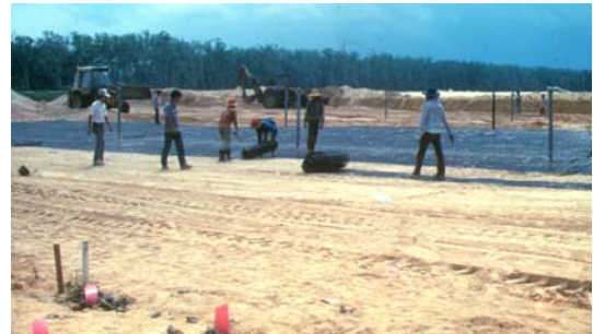
Figure 4e Muar Flat Trial 1987, laying of geogrids
