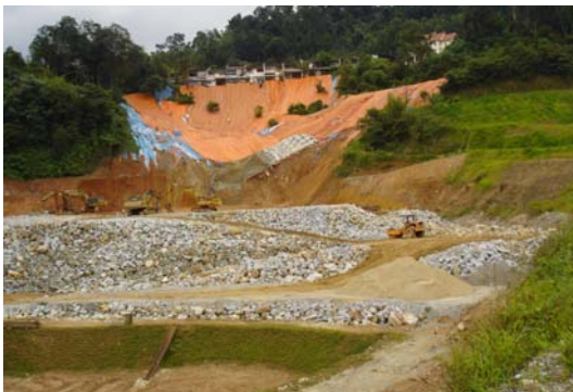
Figure 20h Construction of lower rock fill embankment
