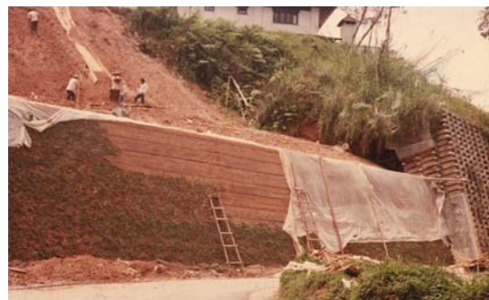
Figure 2c Slope rehabilitation in progress, 1987
