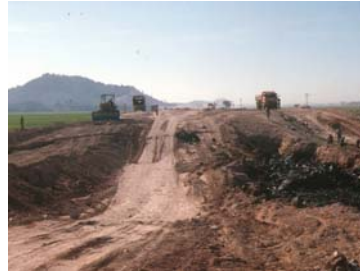
Figure 4b Excavation in embankment
