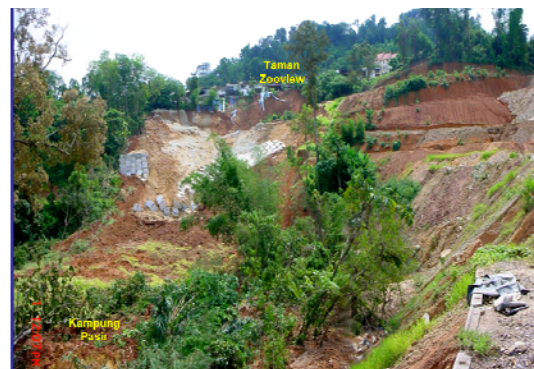
Figure 20d Collapse of anchored soil wall 31 st May 2006
