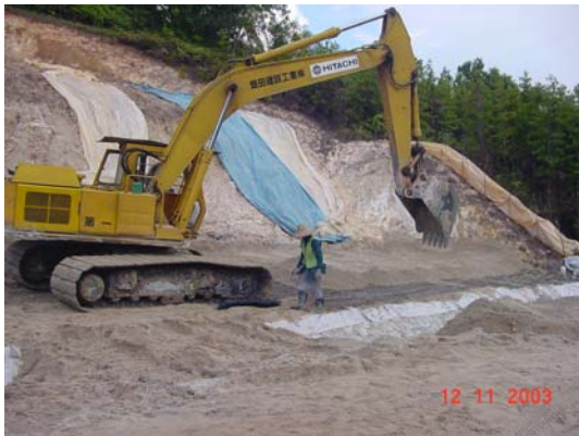
Figure15c Rehabilitation in progress
