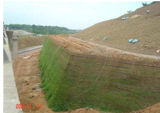
Figure 18e Turfing of geogrid block
