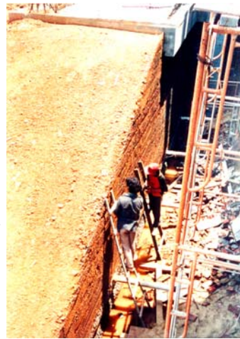
Figure 13b Completed wall
