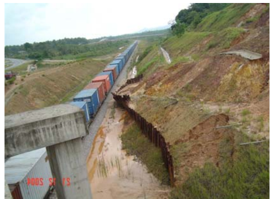
Figure 18b Collapse of slope and sheet pile movement
