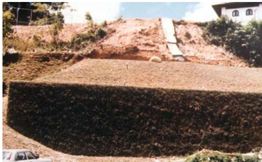
Figure 2d Rehabilitation in progress with upper slope, 1987
