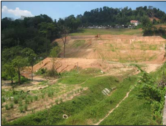
Figure 20n Rehabilitated slope on completion.
