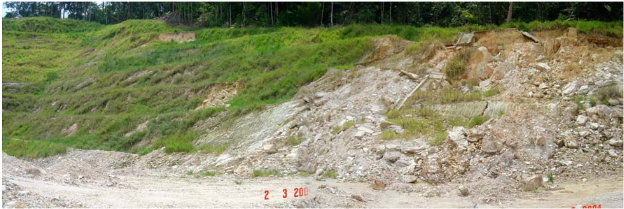
Figure 21a View of slope failure in March 2004.
