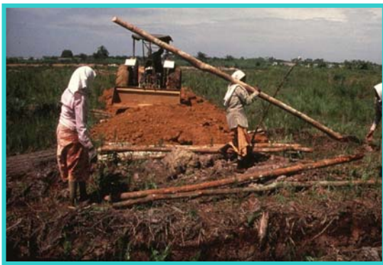
Figure 6 Laying of bakau mats for soft ground stabilization
