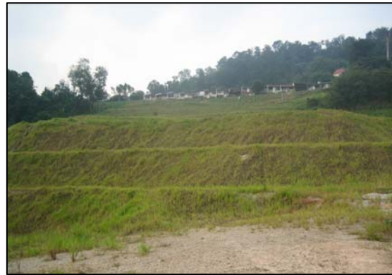
Figure 20p Rehabilitated slope with turf established
