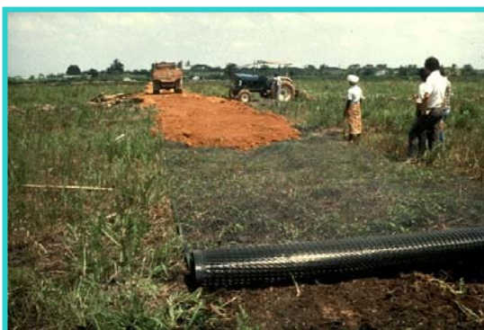
Figure 7 Laying of geogrid in soft ground
