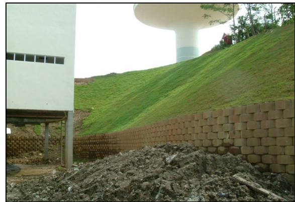
Figure16d Rehabilitated slope
