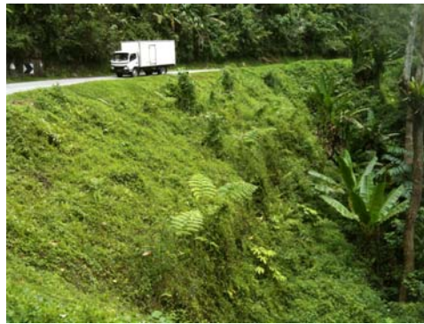
Figure 19e Recent view of rehabilitated slope
