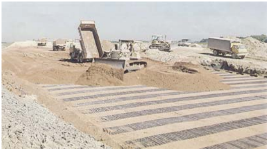
Figure 4d Laying of SR2 uniaxial geogrid
