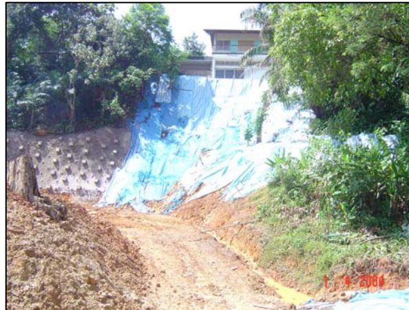
Figure17a Collapse of cut slope during soil nailing
