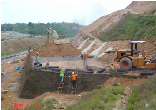
Figure 18d Construction of geogrid block on stabilized base
