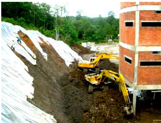
Figure 16c Removal of debris and cutting back of slope
