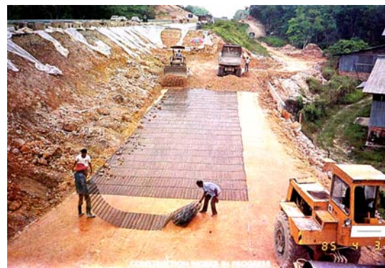
Figure 3b Rehabilitation in progress; laying of geogrid
