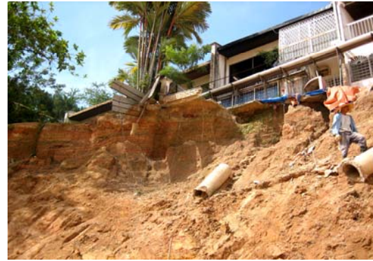
Figure 20m Condition of backyard before rehabilitation
