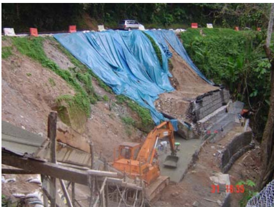
Figure 19c View of slope on rehabilitation
