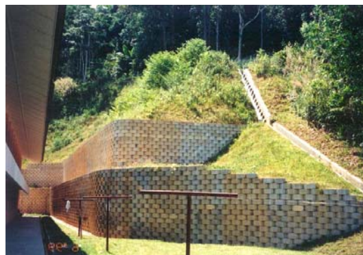
Figure 14c View of Rehabilitated Slope
