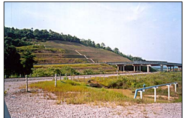
Figure 18g Overall view of rehabilitated slope
