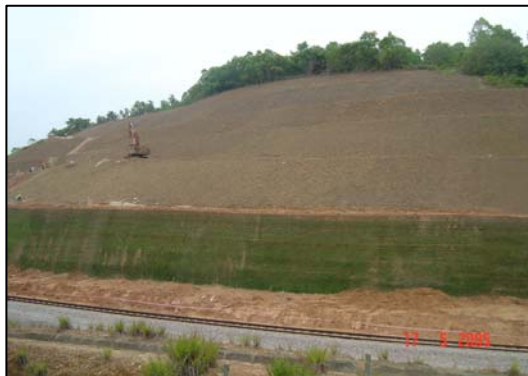
Figure 18f View of rehabilitated slope
