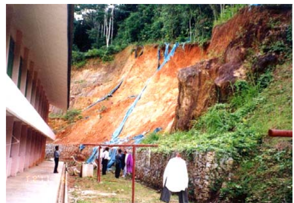
Figure 14a Slope failure above toe wall close to the school block
