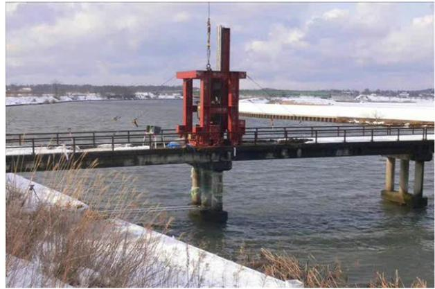
Photo 4 SH devices placed on the bridge
