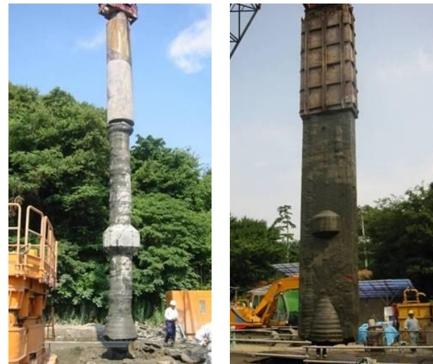
(a) Nodular cast-in-place concrete pile
