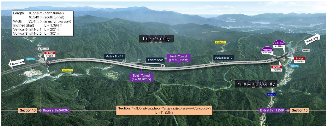
Figure 2 Aerial view of Inje Tunnel
