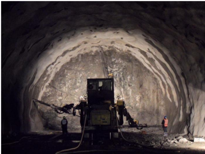
Figure 37 Drilling works for the blasting
