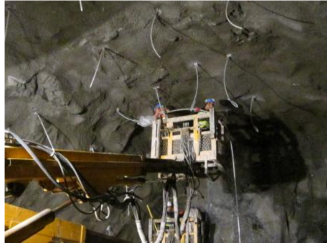
Figure 39 Rock bolt installations
