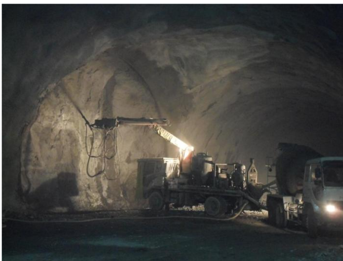
Figure 38 Shotcrete placements after the blasting
