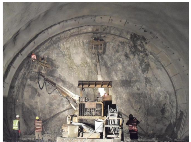
Figure 40 Steel rib (Lattice girder) installations
