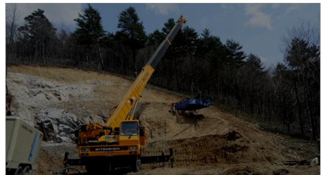
(a) Soil nailing
