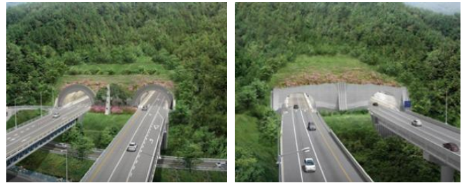
Figure 25 Portals at both ends of the tunnel
