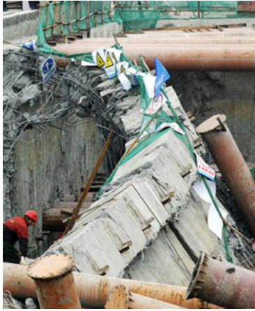
Figure 15 Brackets of pipe struts
