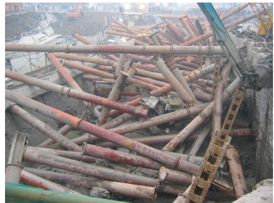
Figure 14 The messy struts after the collapse
