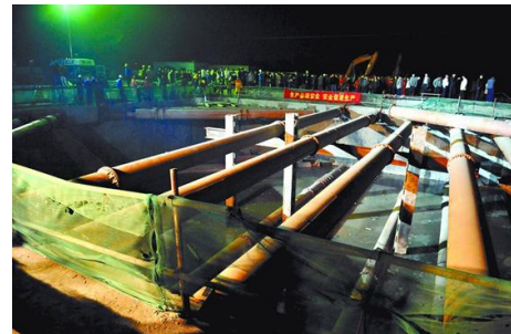
Figure 19 Pipe struts and their vertical support structure
