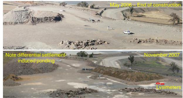
Figure 16 Differential settlement and hard-panning of surface of Cadia's trial waste rock dump over time, causing internal runoff and concentrated ponding
