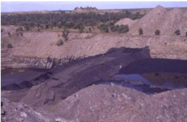
Figure 7 Typical in-pit washery waste storage (tailings behind a coarse reject bund) at a black coal mine
