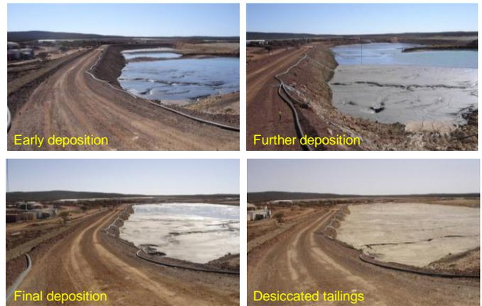
Figure 30 Cosmos tailings deposition and desiccation cycles
