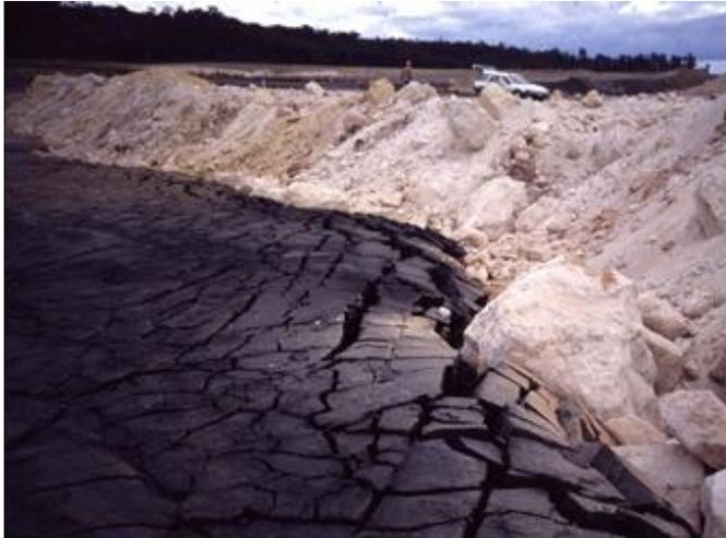
Figure 33 Bow-wave failure of crusted coal mine tailings due to rapid placement of an excessive thickness of cover material
