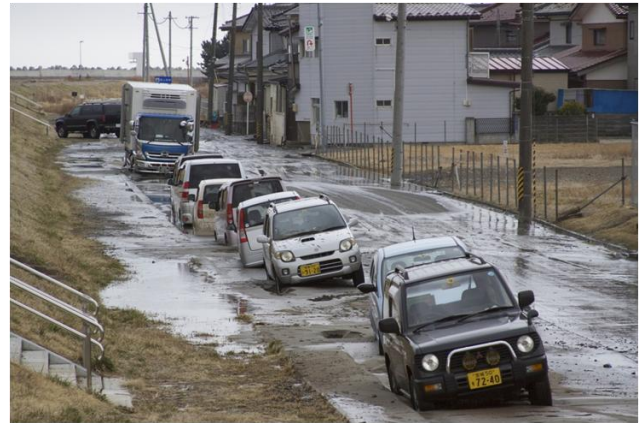
Figure 9 Liquefaction under the Natori River levee in 2011 (courtesy of Tohoku Regional Development Bureau, Ministry of Land, Infrastructure, Transport and Tourism)
