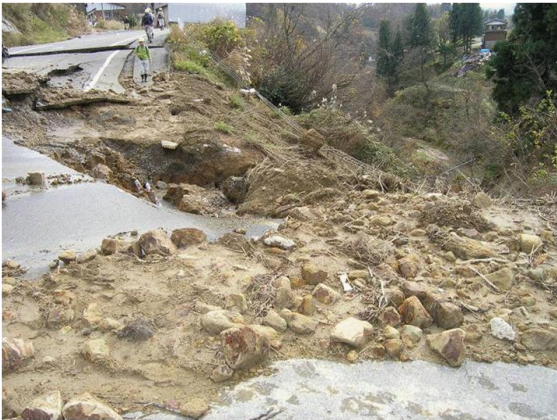
Figure 12 Earthquake-induced failure of road embankment made of crushed mudstone
