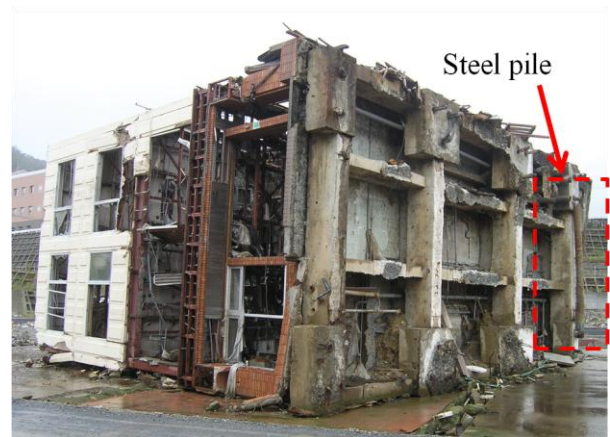
Figure 10 Base of tsunami-overturned building with pile foundation in Onagawa Township
