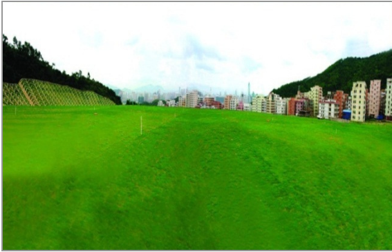
Figure 6 A landfill final capping with vegetation in China
