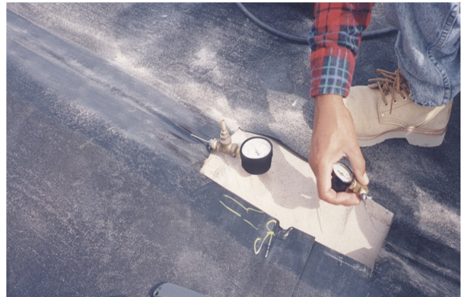
Figure 8 Non-destructive air pressure test is in progress at site
