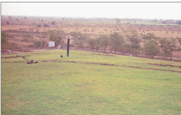
Figure 7 A completed landfill capping system in Western India
