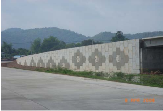
Figure 3 Application of BRE wall for highway structure in Suraburee Interchange project.
