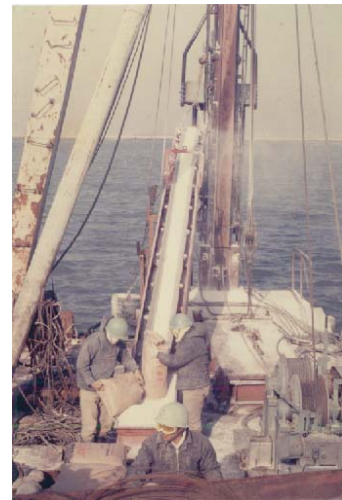
Figure 2 First full-scale test at offshore Haneda in the early 1970s (courtesy of Port and Airport Research Institute)
