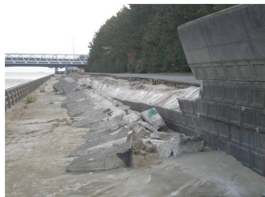
(c) River embankment without improvement
