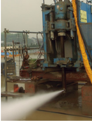
(c) High pressure injection method
