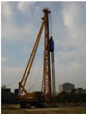
Figure 16 Typical CDM machine for on-land work in operation
