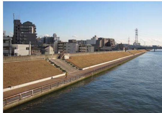
(b) River embankment at the Naka River
