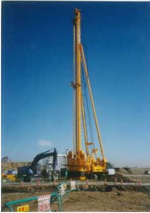
(a) Dry mixing method for on-land works
