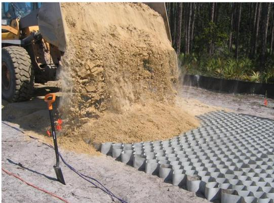
Figure 1 Filling of sand into geocell
