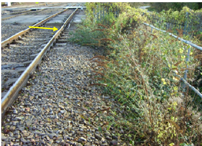
Figure 1 Typical transition fault (indicated) at the bridge interface
