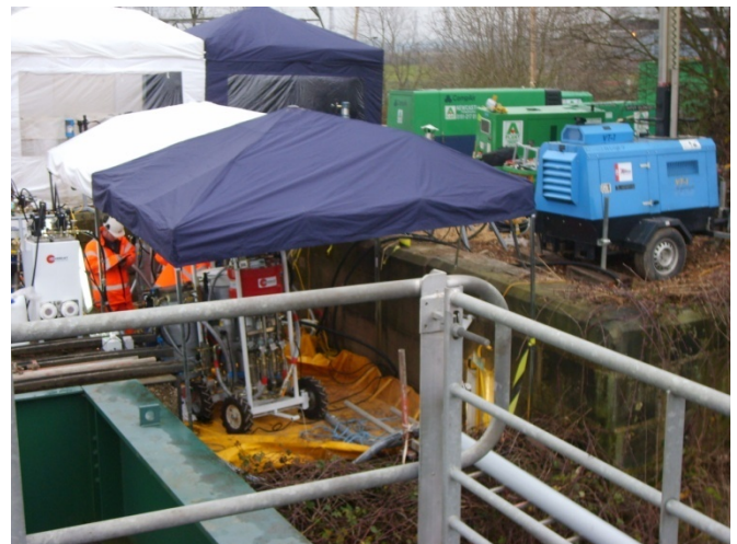
Figure 12 Typical pumping unit (pneumatic variant shown)
