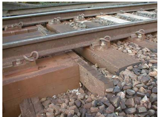
Figure 2 Hanging sleepers at bridge interface (from floating to fixed track geometry)
