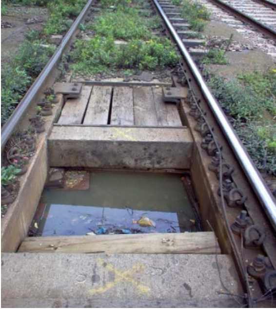
Figure 8 Application of long-timber transition beams
