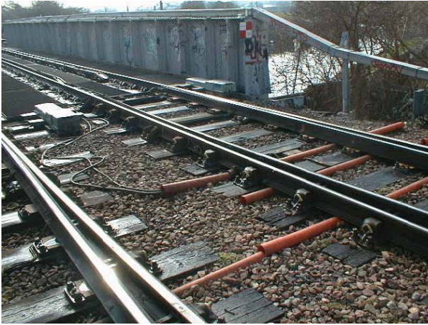
Figure 17 Bridge Transitions Showing Current Location of Point Machines on the Bridge Deck
