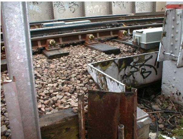
Figure 18 Extension of bridge deck between fixed timbers and floating ballast sections ( lower deck transition slab )
