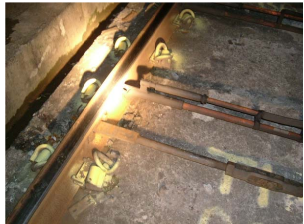
Figure 7 Deterioration of the concrete slab-track due to the development of hanging sleepers in the transition zone
