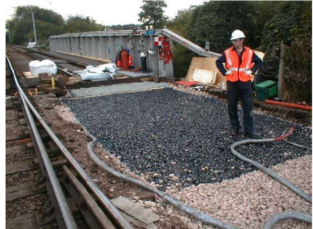
Figure 19 Application of the polyurethane along the bridge transition
