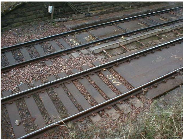
Figure 6 Concrete slab-track transition (transition slab is underneath the transition sleepers)
