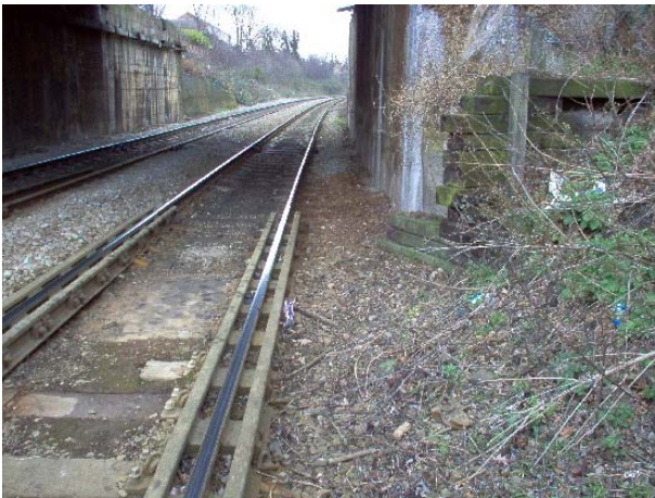
Figure 5 Application of additional rails in the transition zone
