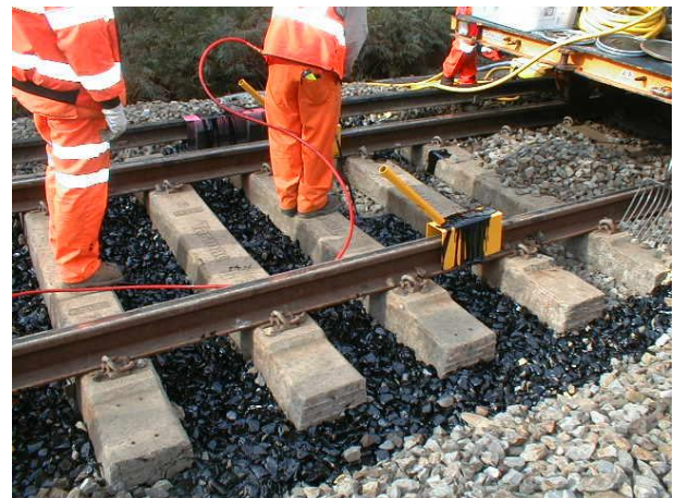
Figure 23 Application of the polymer to form a ladder structure at Worplesdon UK
