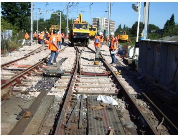
Figure 22 Formation of the upper GeoComposite beams to prevent lateral movement of the sleepers
