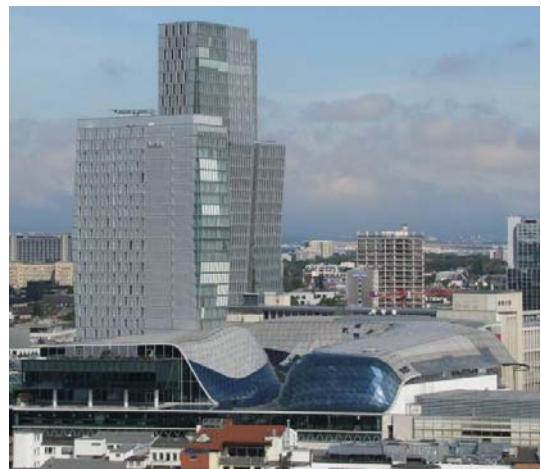
Figure 7 Project "PalaisQuartier", Frankfurt am Main, Germany
