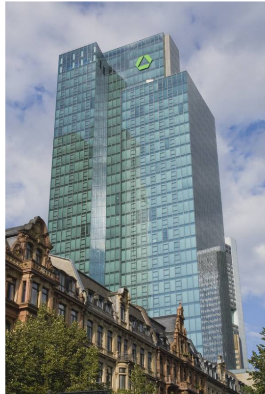
Figure 22 View on the finalised high-rise building
