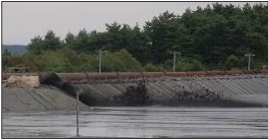
Photo. 3 Aspect of dumping of soil into the landfill site
