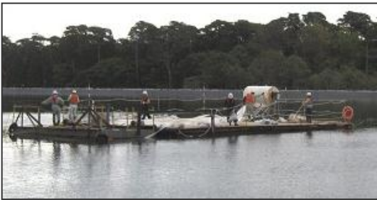
Photo.4 Construction barge for intermediate PBD
