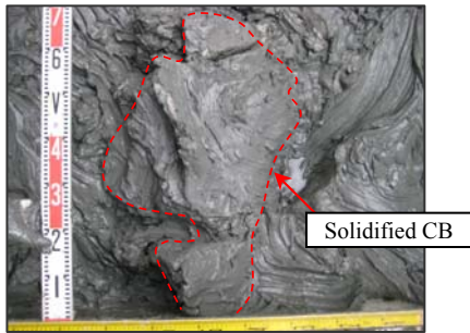
Photo 2 Shape of injected soil after solidification in the ground
