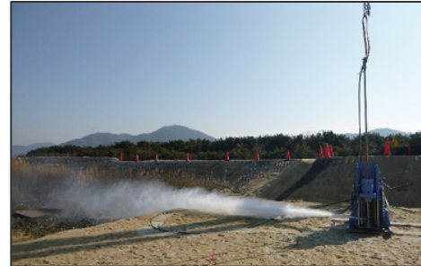
Photo 5 Situation of discharging water jet into the air
