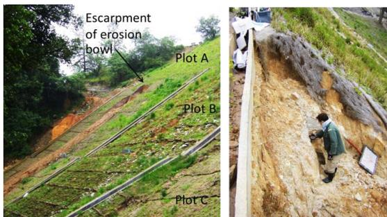
Figure 3 Slope failure and its escarpment at Plot A
