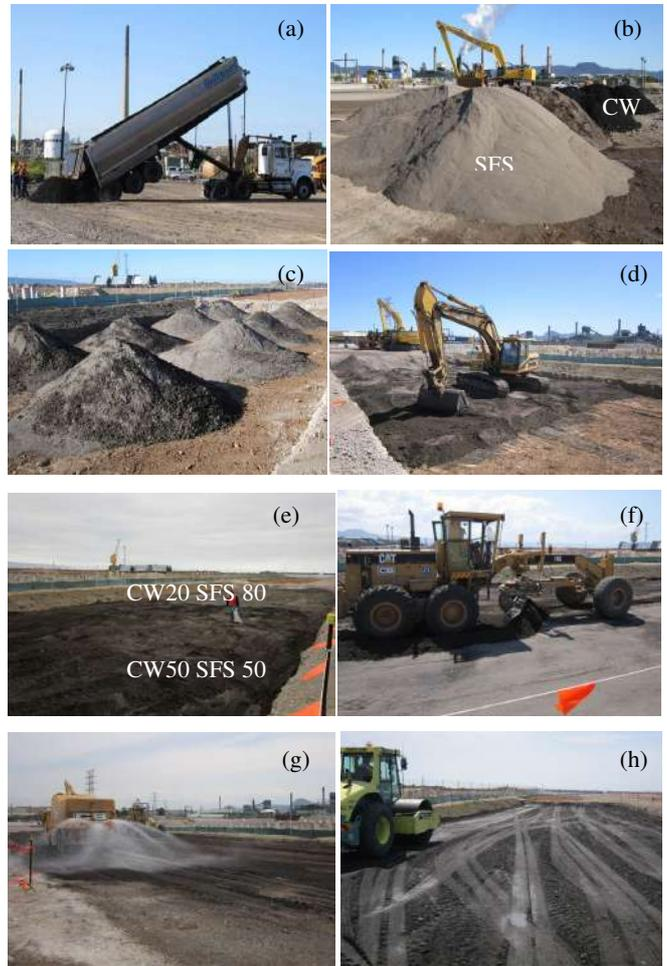
Figure 8 Photos of the field trial (a) arrival of the material on site, (b) stock pile of steel furnace slag and coalwash, (c) mixed materials ready for (d) spreading, (e) sampling prior to compaction, (f) levelling, (g) adding moisture and (h) compaction
