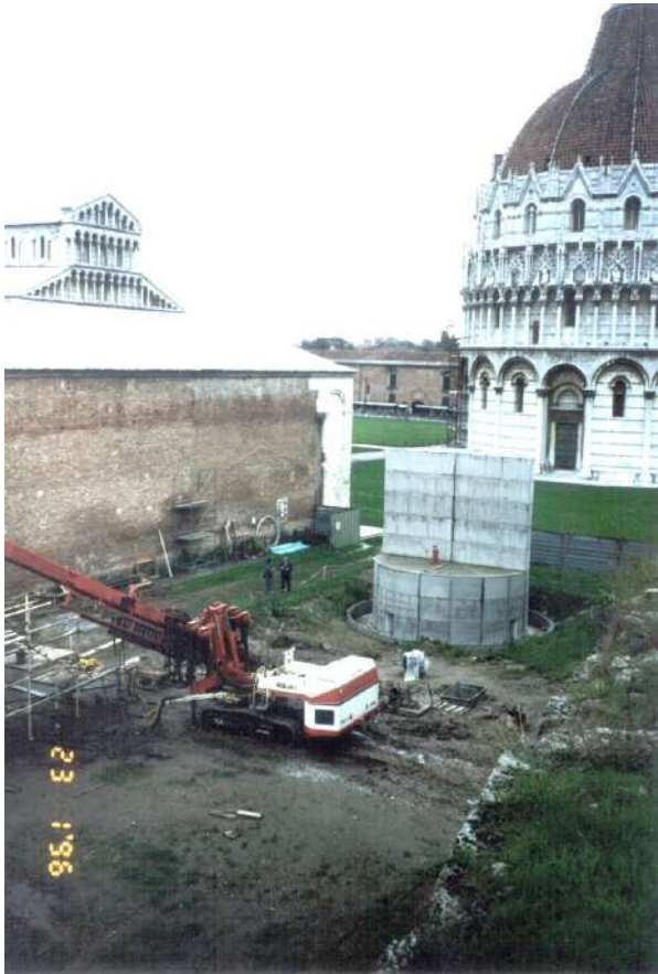
Figure 15 Underexcavation trial field
