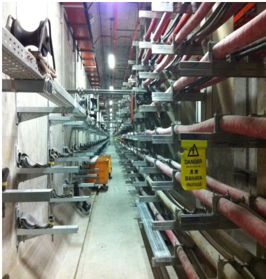
Figure 2 Combined utility cable tunnel
