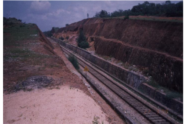
Figure 7 Failures of a deep excavated shedi soil slope (as seen in the far end) and mud pumping along the Konkan railway track.
