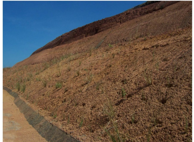
Figure 18 A shedi soil slope along the Konkan railway track Planted with vetiver saplings for erosion control
