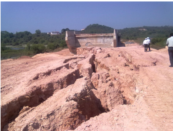
Figure 5 Embankment failure due to poor compaction on untreated soft foundation in lowland environment
