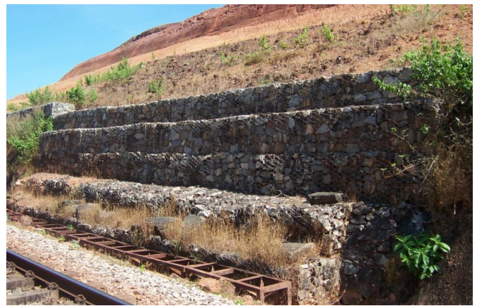
Figure 19 Another section of Konkan railway, where the slope is protected by gabion wall
