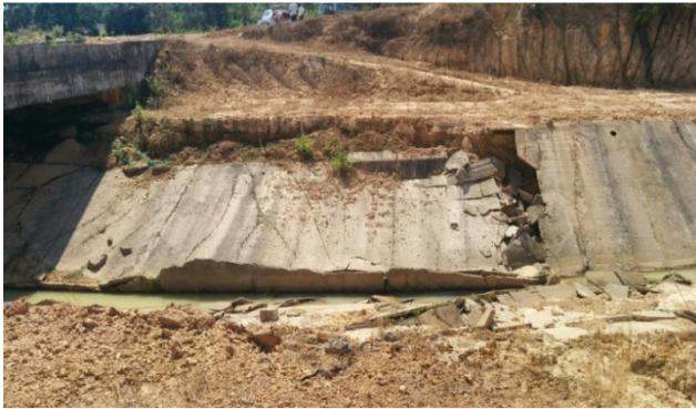
Figure 9 Damages caused to canal lining due to erosion of the lithomargic clay behind it
