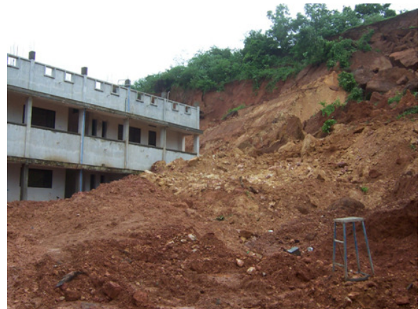
Figure 8 Failure of a steep shedi soil slope adjacent to a building during monsoon season, aided by poor drainage.
