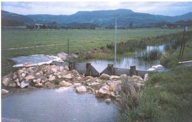
Figure 2 V-notch weir (after Banasiak (2004))
