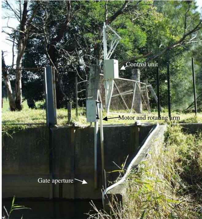
Figure 5 Modified two-way floodgate (Photo courtesy: Glamore (2003))
