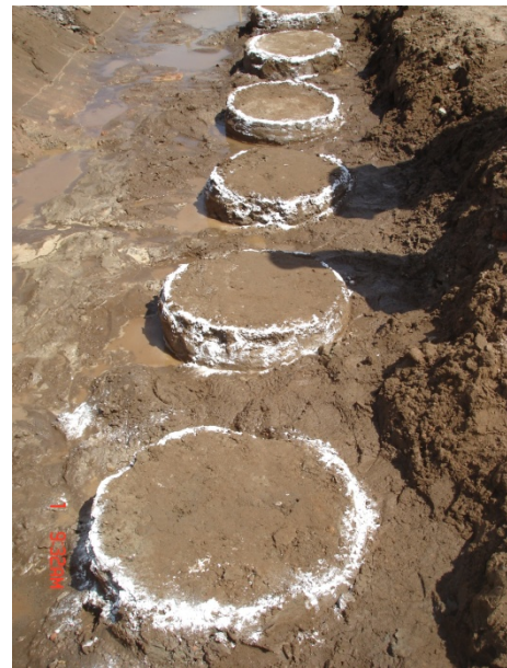
Figure 4 Surface exposure of cement mixed column
