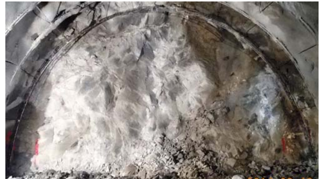
Figure 12 Rock mass condition revealed at the station of 4K+407.5 for the northbound of case tunnel
