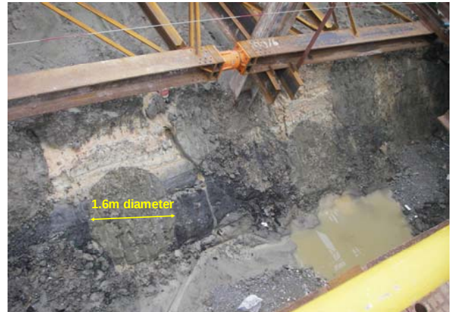
Figure 16 Columns created during withdrawal
