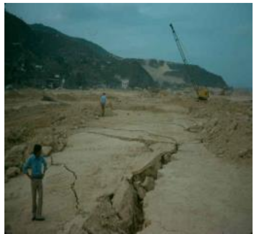
Figure 7 Unstable ground where mud had been displaced
