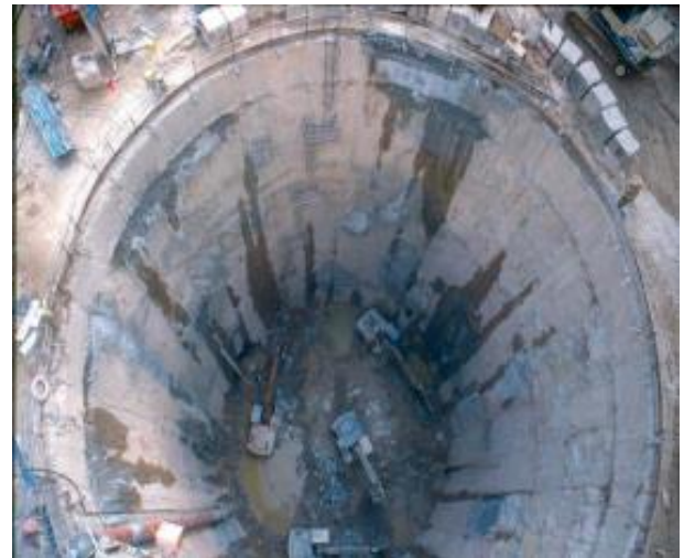
Figure 31 Foundation for one column of an 80 storey building
