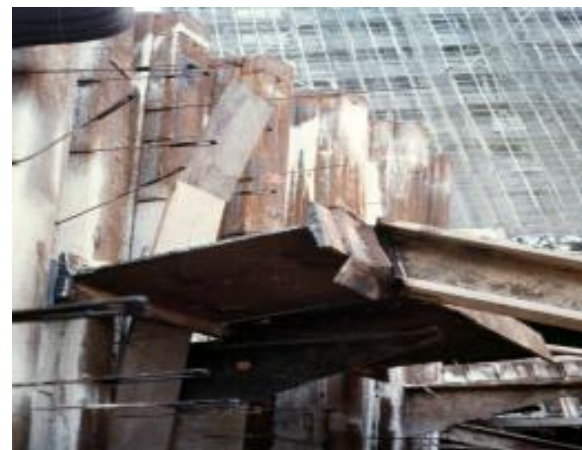
Figure 11 No holding down of waling with inclined strut
