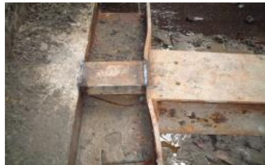
Figure 38 Photo of the changed strut to waler connection
