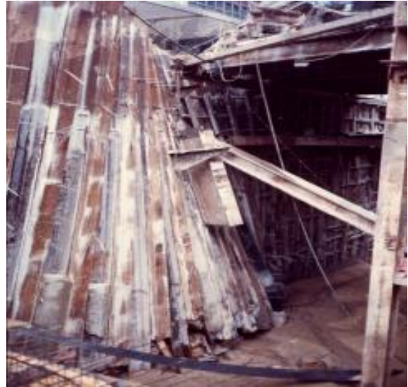
Figure 10 One row of inclined struts and no toe-in for the steel sheet piling
