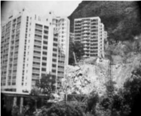
Figure 5 Failure at Po Shan Road which demolished a 12 storey apartment block
