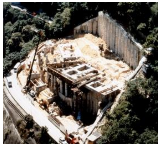
Figure 21 Site formation work in progress on steep site
