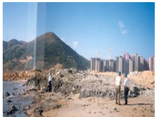
Figure 8 Mud displaced by dumping fill
