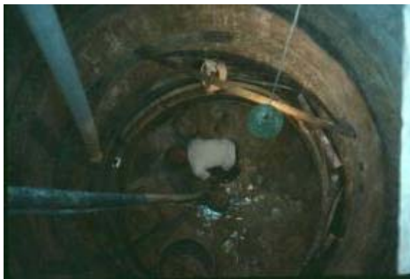
Figure 13 Excavation of a Hand Dug Caisson
