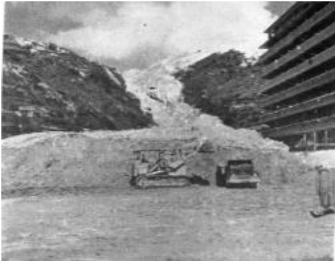
Figure 4 Large volume of debris from a major slope failure
