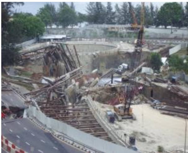
Figure 33 Collapse of cut and cover excavation alongside the Nicoll Highway, Singapore
