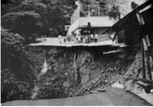
Figure 3 Collapsed road due to landslide
