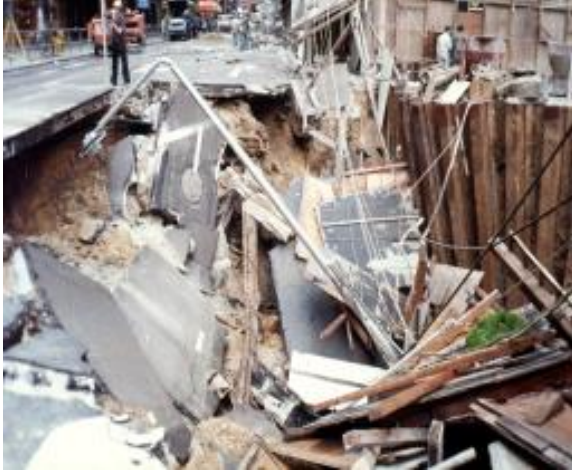
Figure 9 Collapse alongside excavation for a basement in Central in 1981
