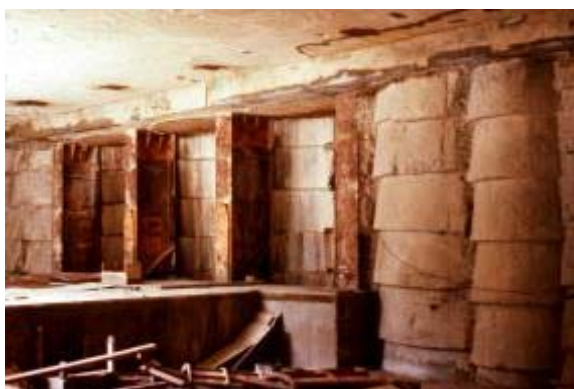
Figure 14 Underground station walls constructed by hand dug caissons
