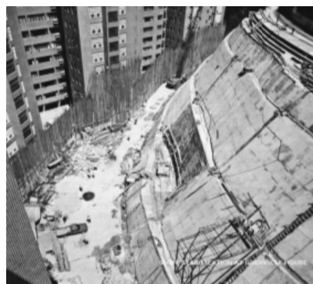
Figure 17 Installation of horizontal drains in steep slope
