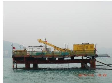
Photo 3 Completed temporary working platform
