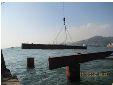
Photo 1 Erection of steel beams on top of piles
