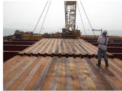
Photo 2 Erection of steel decking
