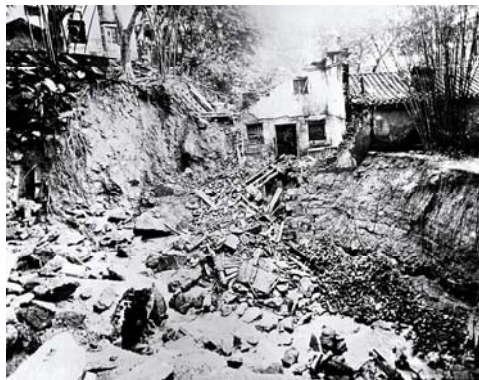
Figure 1 Landslide occurred in May 1889 in Glenealy, Central
