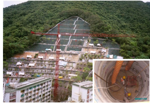
(a) Construction of hand-dug caissons at Sai Wan Estate, Hong Kong
