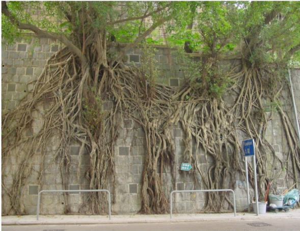
Figure 6 Upgrading of an old masonry wall by soil nails
