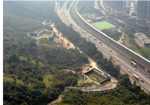
Figure 7 Concrete barriers at the toe of a natural hillside
