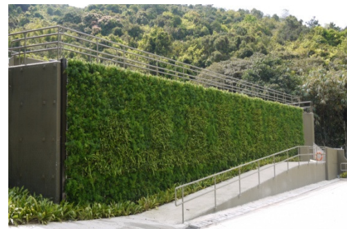
(a) Vertical greening on a concrete barrier
