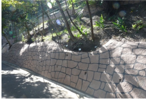
(a) Masonry-like finish on hard slope cover
