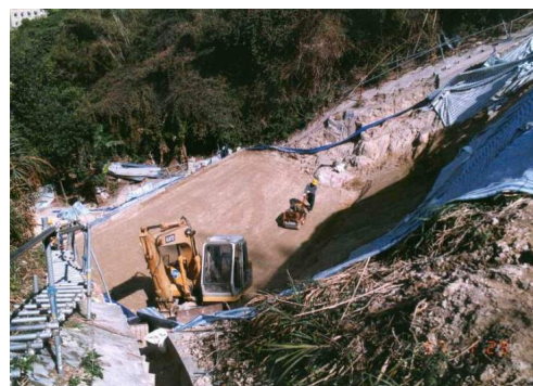
Figure 4 Re-compaction of existing fill
