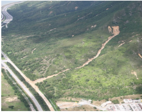
(a) 2008 landslide at Yu Tung Road, Lantau
