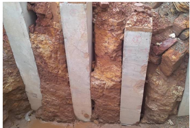
Figure 6 Reinforced concrete square piles in non-backfilled pre-bored holes at weathered meta-sedimentary formation
