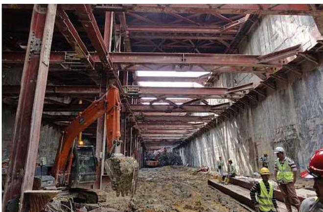
Figure 17 Bottom up excavation at the Merdeka Station
