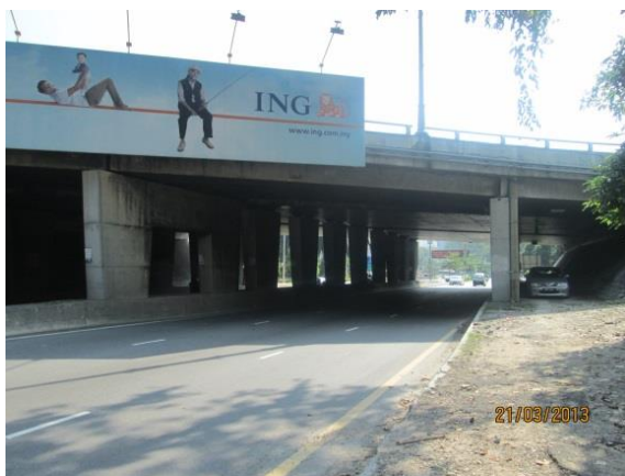
Figure 7 Photo of Flyover
