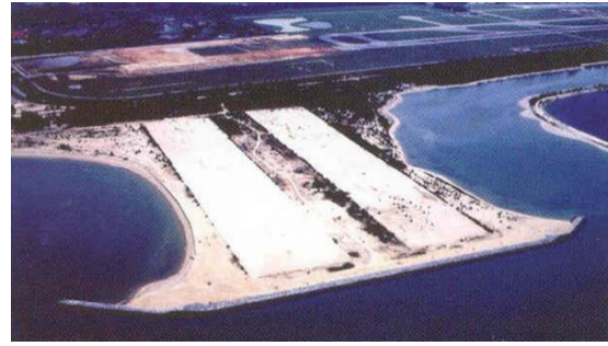
Figure 8 Field trial of the layered clay-sand reclamation method at Changi, Singapore
