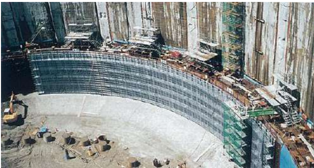
Figure 51 Installation of a block hoop at the depth of -28m
