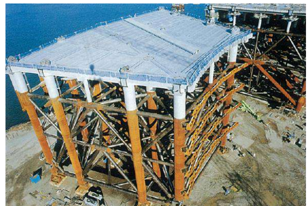
Figure 47 Unit of jacket frame sitting on the assembling yard
