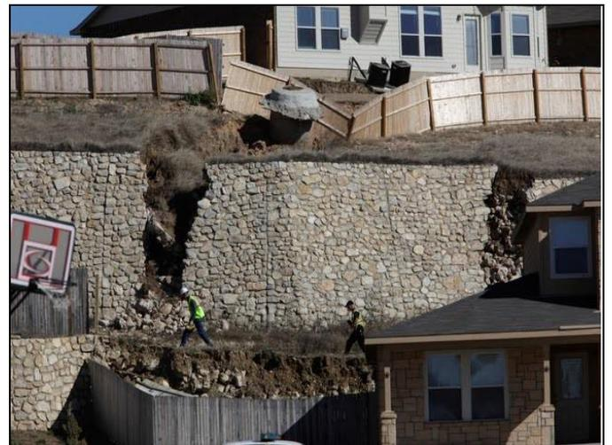
Figure 1 The Collapse of a Retaining Wall that has a Clay Backfill (Dave, 2010)
