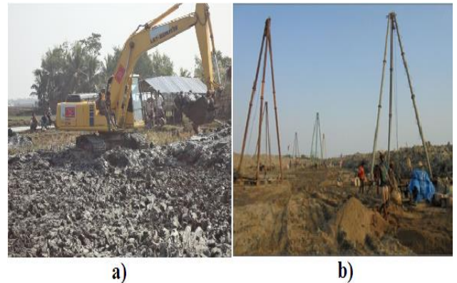
Figure 6 Figure a) shows that removing of soft clay before construction of the VSD pile and b) the construction of the VSD
