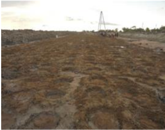
Figure 4 Figure shows square pattern of VSD after completion of the work
